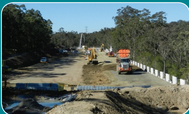
The Hunter Expressway project underway
