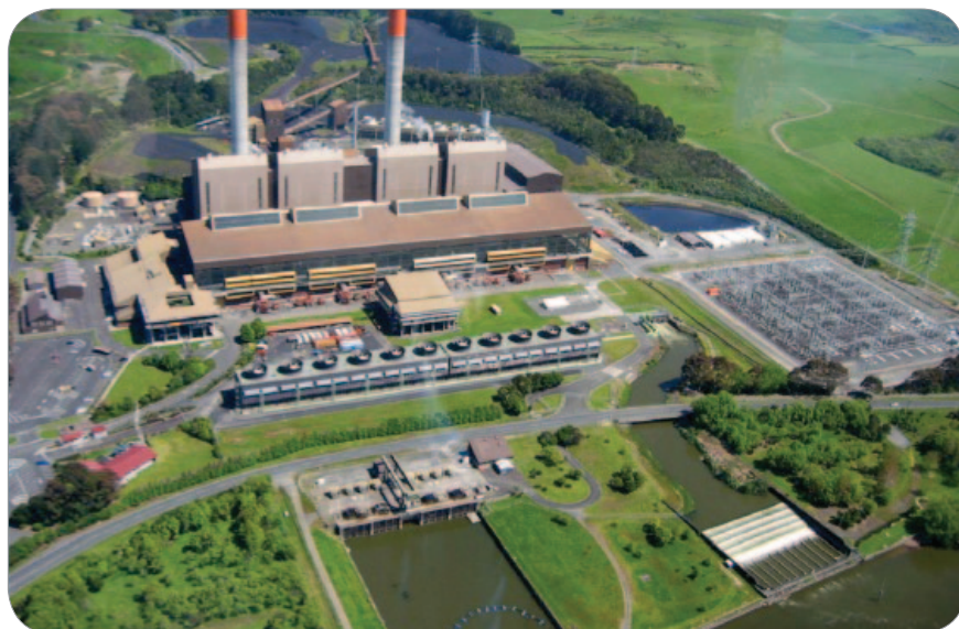
Huntly Power Station from above
