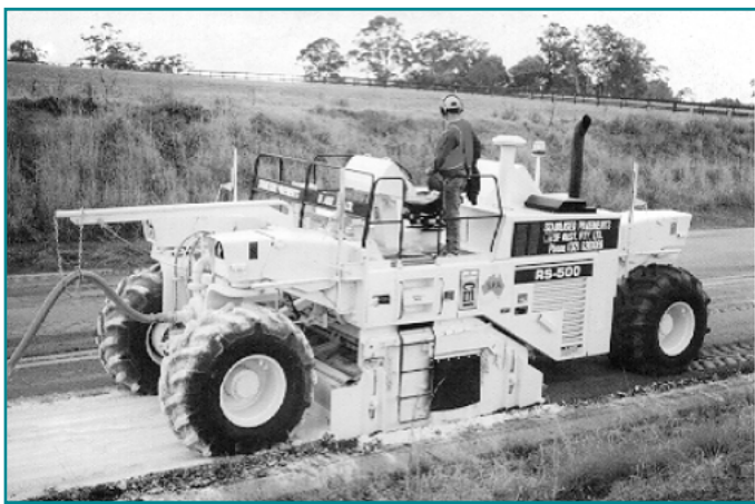
Fig. 2 Example of a Deep Lift Stabilise (7)
