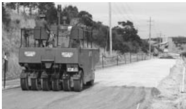
Road construction at Eraring Power Station
