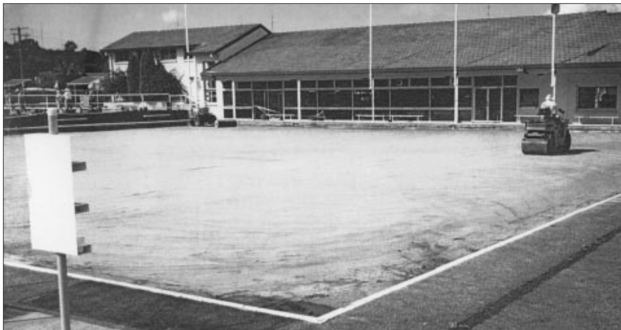
Boolaroo, NSW bowling club used a base of Eraring ROS ash under a synthetic playing surface.
