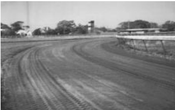
A further project for Eraring ROS ash was the preparation of a training track for Newcastle Jockey Club at Broadmeadow. Similar tracks are in service at Coffs Harbour, Wyong and Randwick.
