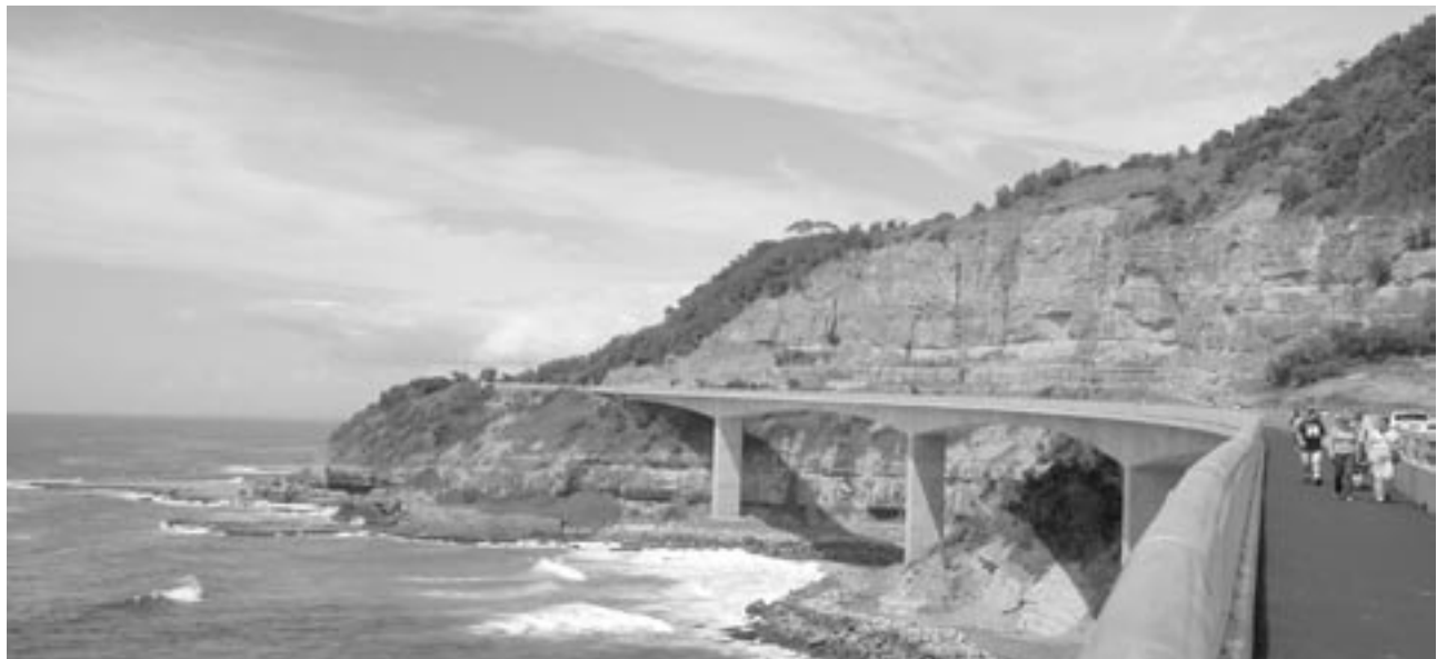
Image 2: LHD Pedestrian Walkway
