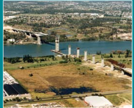
Above (fig. 1): Original Gateway under construction
