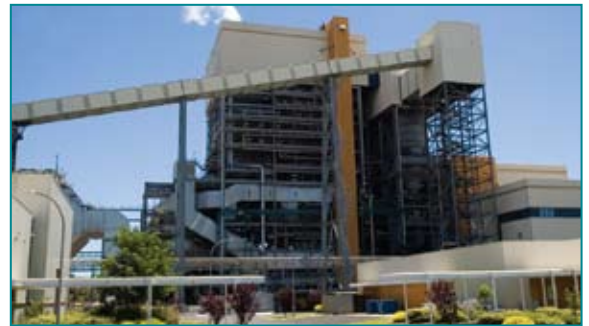
Above: Collie Power Station
