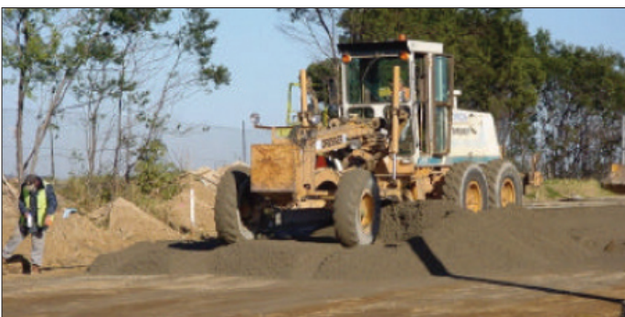
Fig. 1: Grader used to Spread RCC (3)
