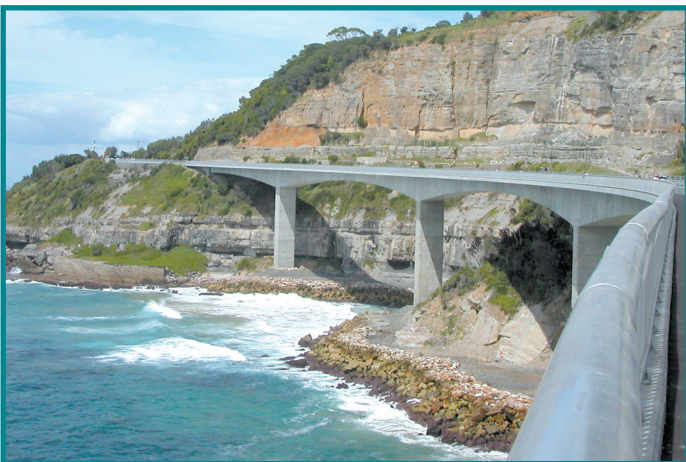
Image 1 - Sea Cliff Bridge . Concretes used in marine environments must be adequately designed to minimise destruction by corrosion
