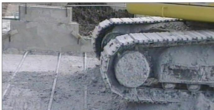
Fig. 3: Spreading and Compaction of Fly Ash - Mt Piper Power Station Reinforced Soil Wall<sup>(9)</sup>
