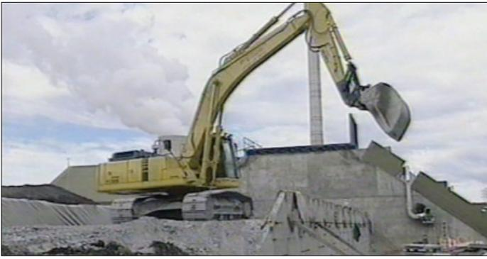
**Fig. 1:** Fly ash as a Structural Fill - Earth Reinforced Wall - Mt Piper Power Station <sup>(9)</sup>
