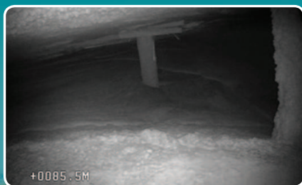
Infill paste flowing down old roadway – photo from remote borehole video camera
