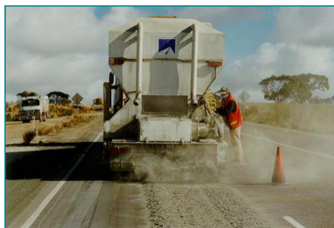
Fig. 3 FA and lime blend, South Australia (10)
