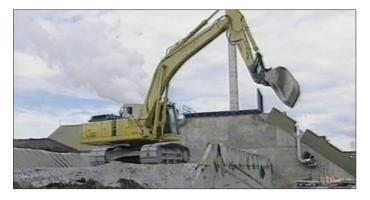
Fig. 1: Fly ash as a Structural Fill - Earth Reinforced Wall -Mt Piper Power Station (<sup>9</sup>)
